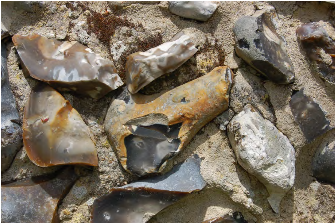
Picture 1.6 Field gathered flint used in the wall surrounding Little Easton Church.
