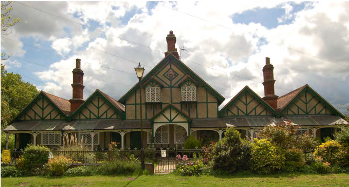
Picture 1.12 Church Row, set back form the road behind highly decorative railings is a building of great charm.
