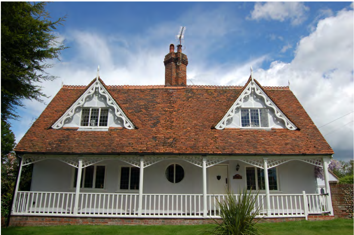
Picture 1.13 Church Lodge with its elegant 19th century verandah and pierced bargeboards makes a bold statement in the street scene.
