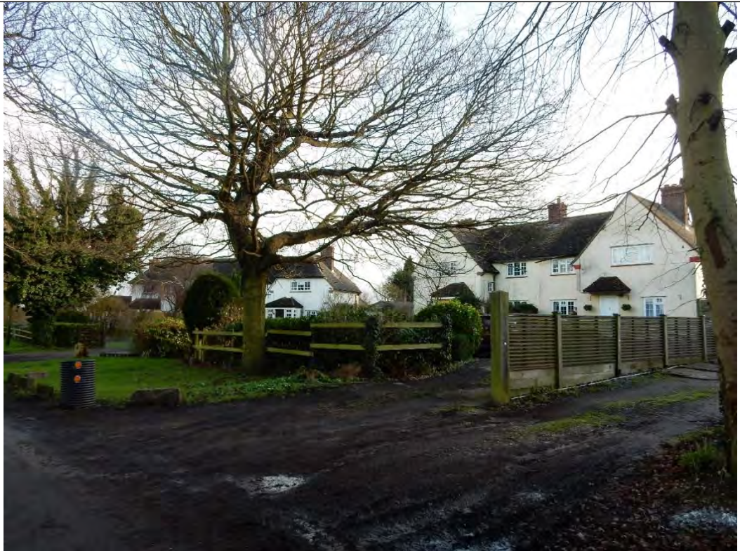
Photograph 222: Examples of housing development on the west side of High Easter Road.
