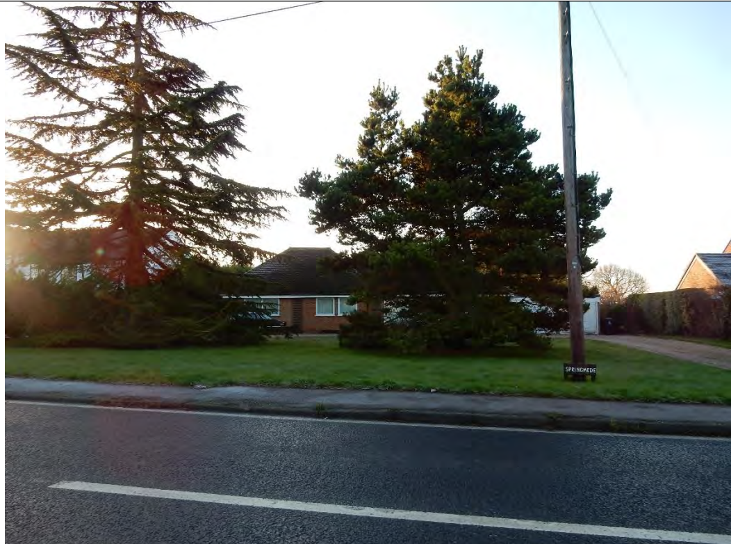
Photograph 116: View of residential ribbon development on Sawbridgeworth Road at the north of the land parcel.
