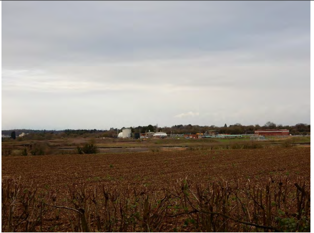
Photograph 083: View of Jenkins Lane sewage works from Church Lane (looking north).
