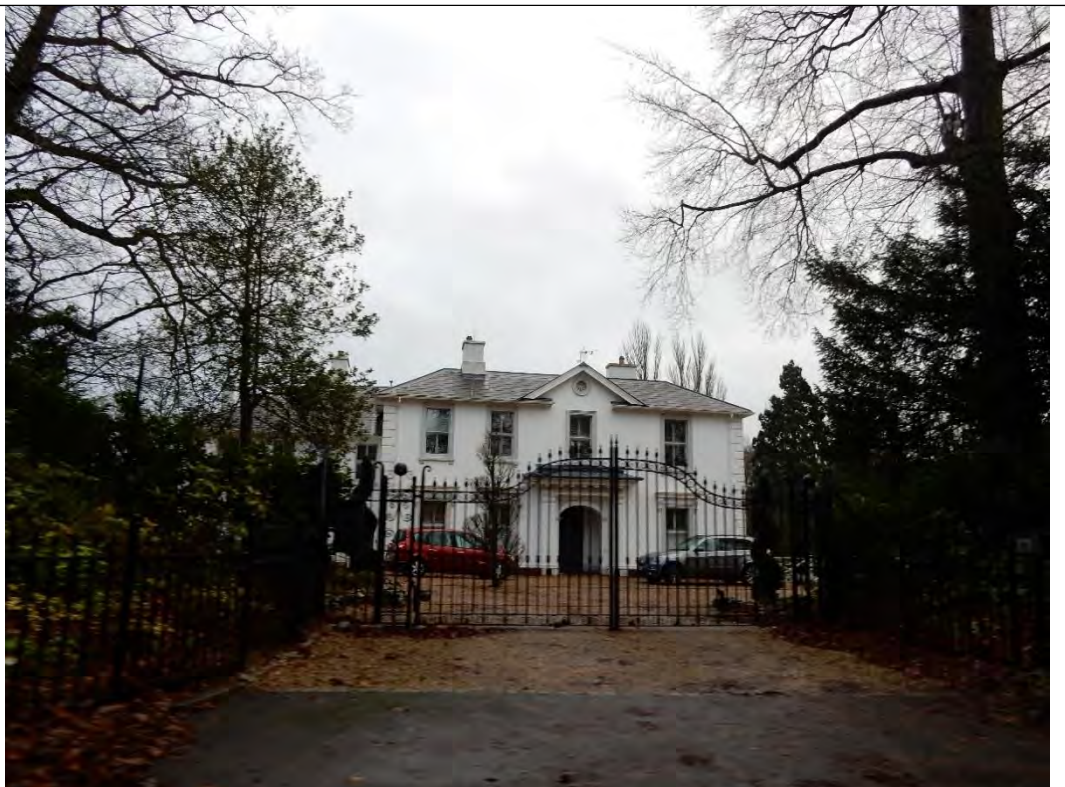
Photograph 040: View of Brookland Manor House on Pines Hill in the centre of the land parcel.
