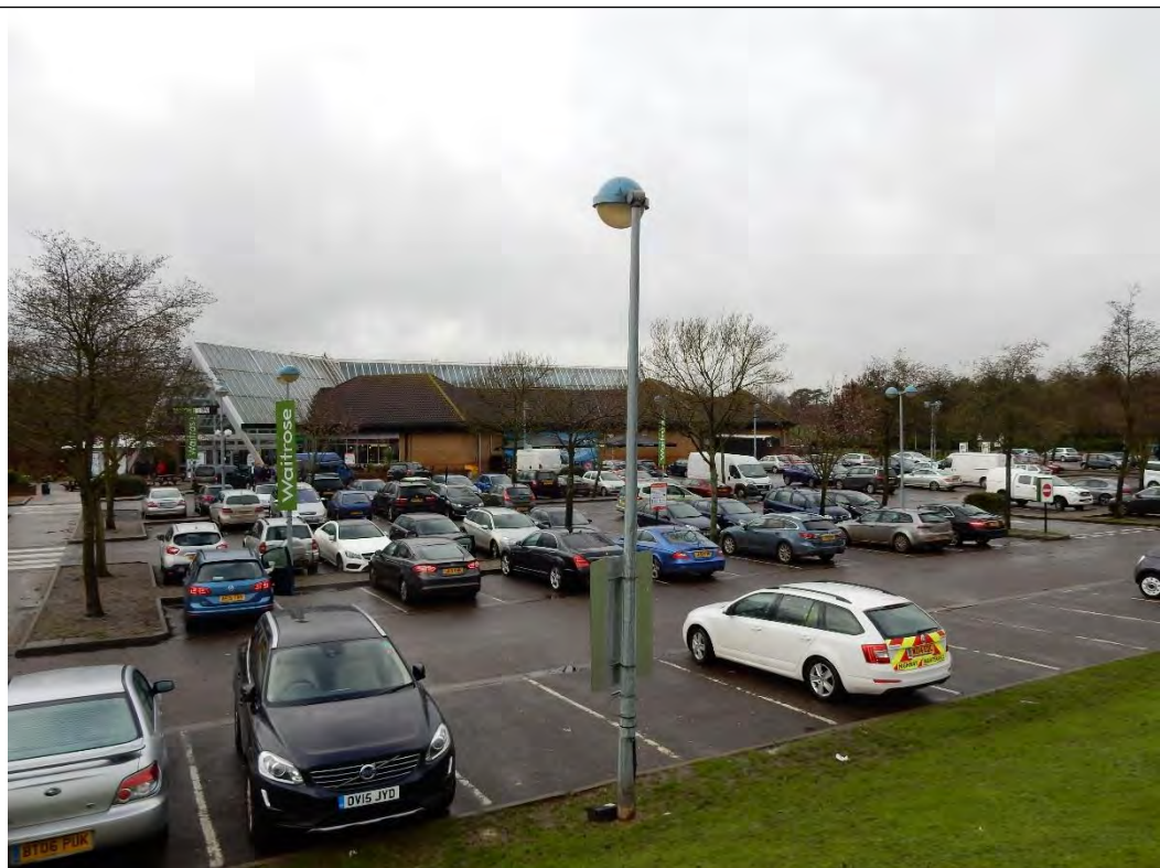
Photograph 063: View looking north-west of Birchanger Green Services, showing high proportion of built-form.
