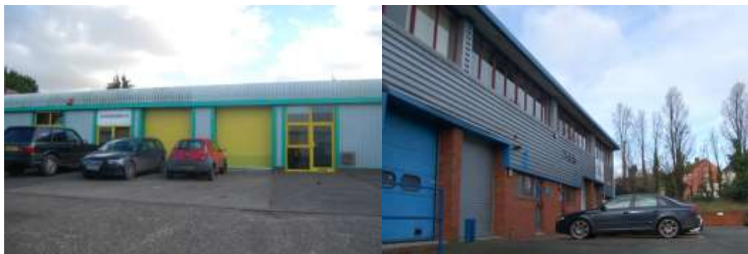
Source: AECOM 2016. Locations from left to right: Golds Business Park (C3) and Saffron Walden Business Centre (C18)
