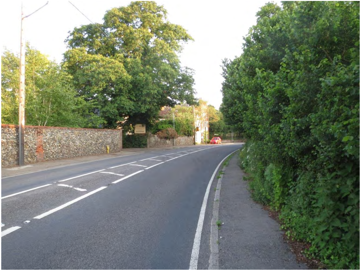
View 19 View westwards along Newmarket Road showing the curve of the road as it echoes the Roman town walls
