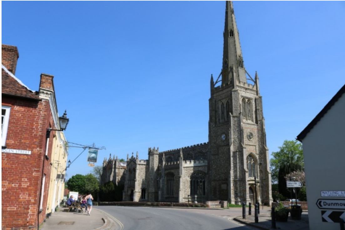
Plate 1: The grade I listed Church of St John the Baptist
