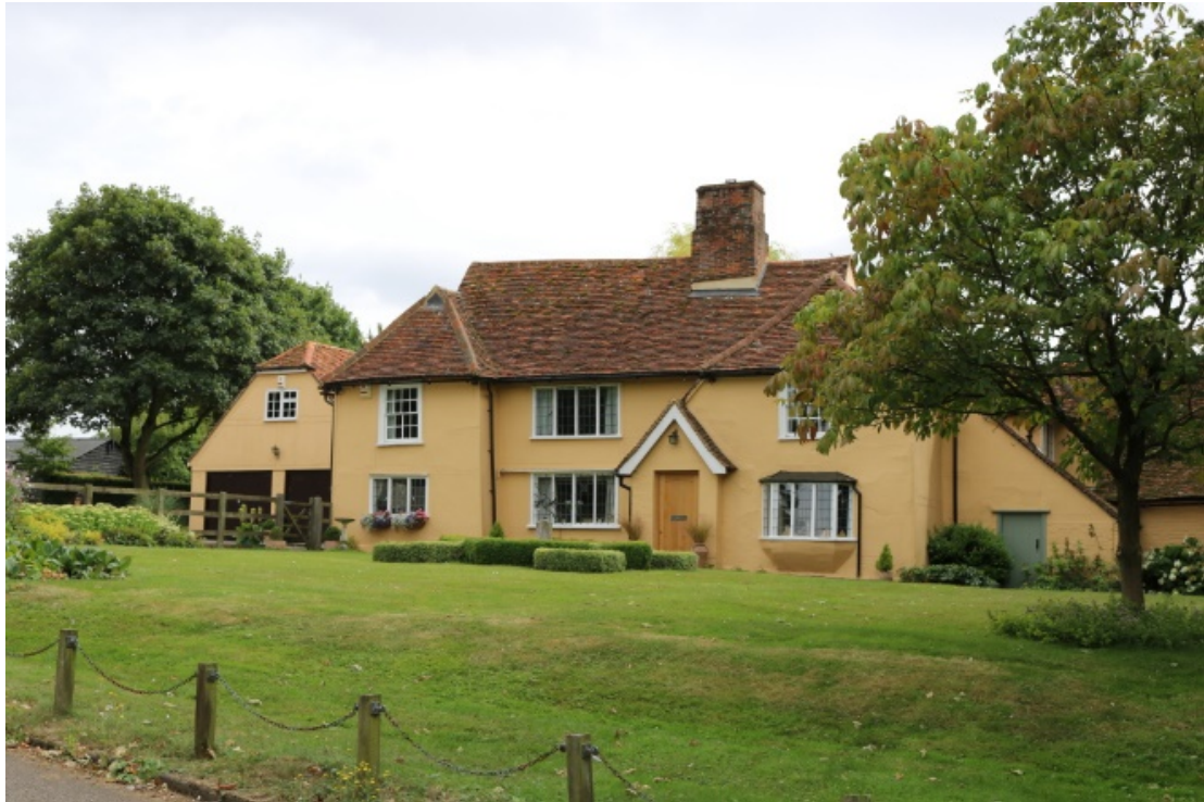
Plate 29: The north façade of the grade II listed Claypits Farmhouse, seen from the existing private access drive
