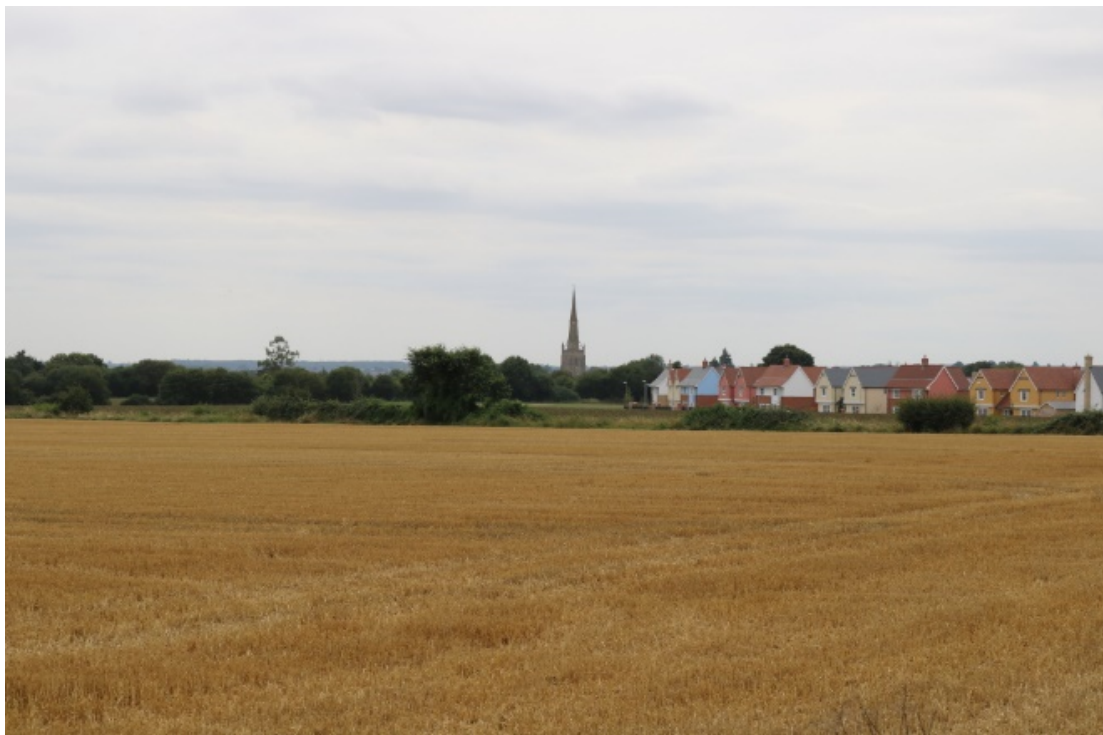
Plate 22: View from Sampford Road across Site 04 towards the parish church with the Thatcher's Grange development to the right
