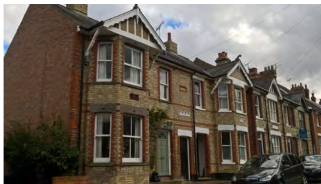
Picture 1.37 No.s 46 - 52 Fairycroft Road
