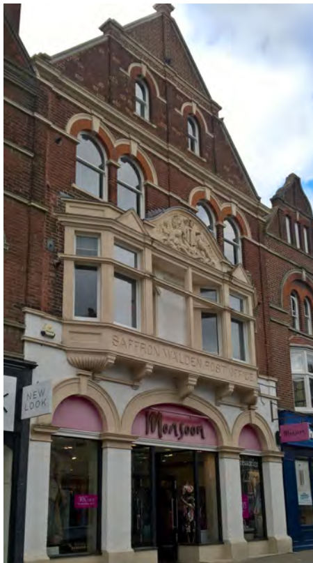
Picture 1.20 Numbers 8-16 King Street, particularly fine architectural detailing
