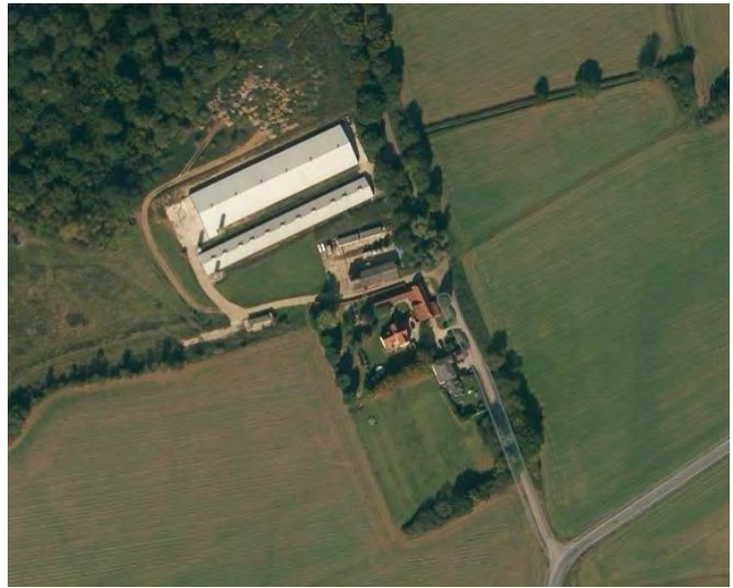
Aerial view of Badcocks Farm
