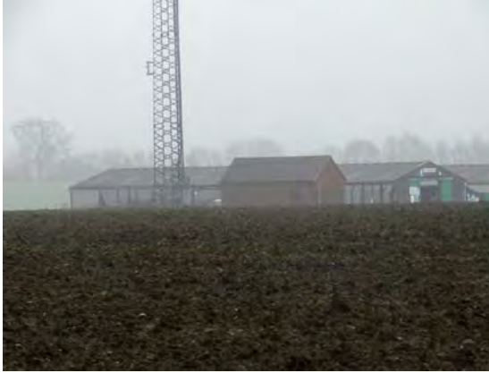
Modern buildings and mast within Deer Park with south east park boundary beyond
