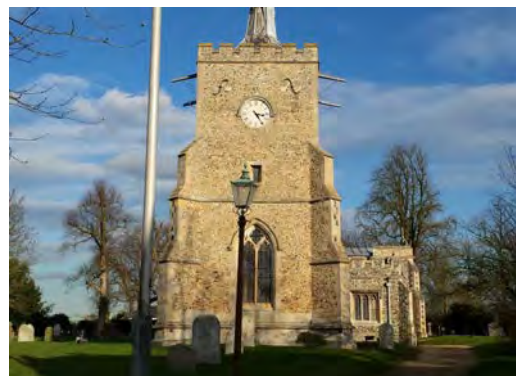
Ickleton Church on the east side of the Conservation Area
