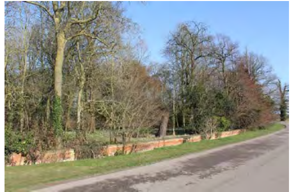
Easton Lodge southern boundary
