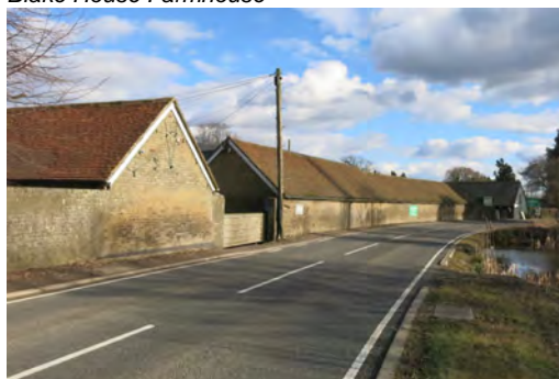
Farm outbuilding range
