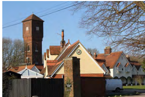
View of Water Tower and Terrace, right
