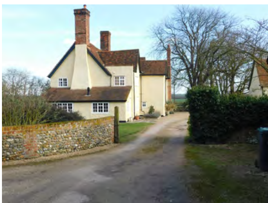
Park Farm House viewed from the north west
