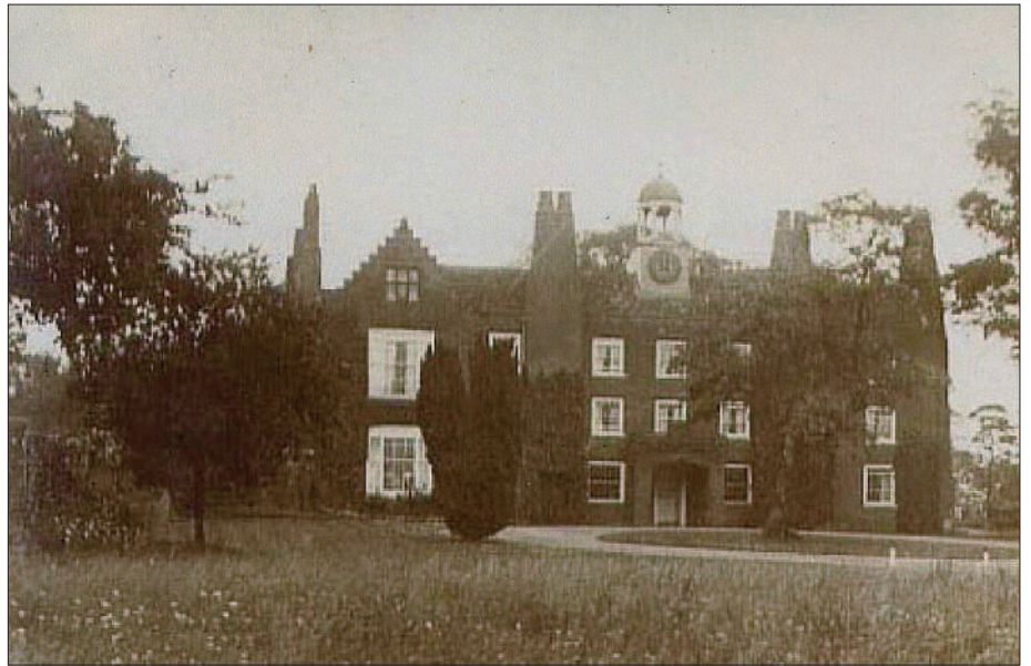
Lofts Hall before the fire in 1934.
