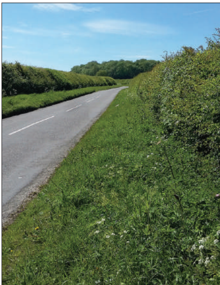
Protected lane No.15 from B1039 towards Bridge Green.
